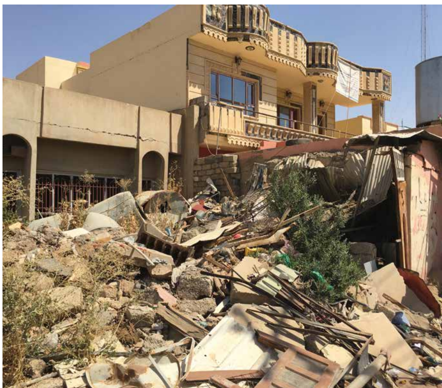
Malteser International is helping to restore 2,200 houses in the Nineveh Plains of northern Iraq.
