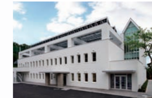
北側外観 North Elevation
