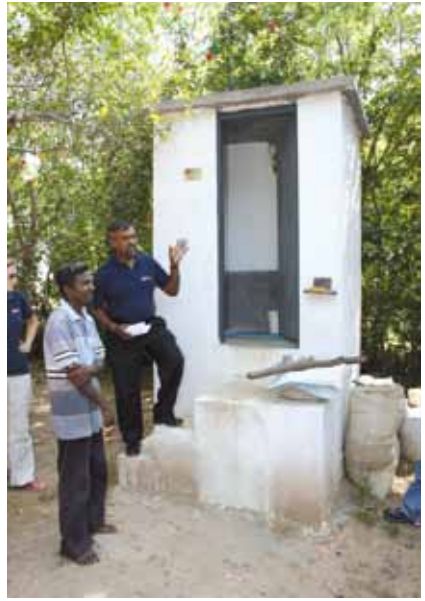
Eco-friendly solution also in dry seasons: compost latrines work without water, faeces are collected and can be composted again for the fields.
