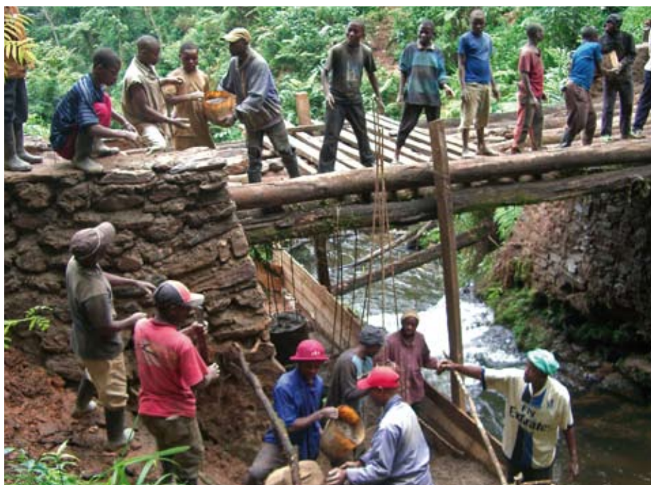
DR Congo: Reconstruction of streets and bridges in Mulungu/South Kivu
