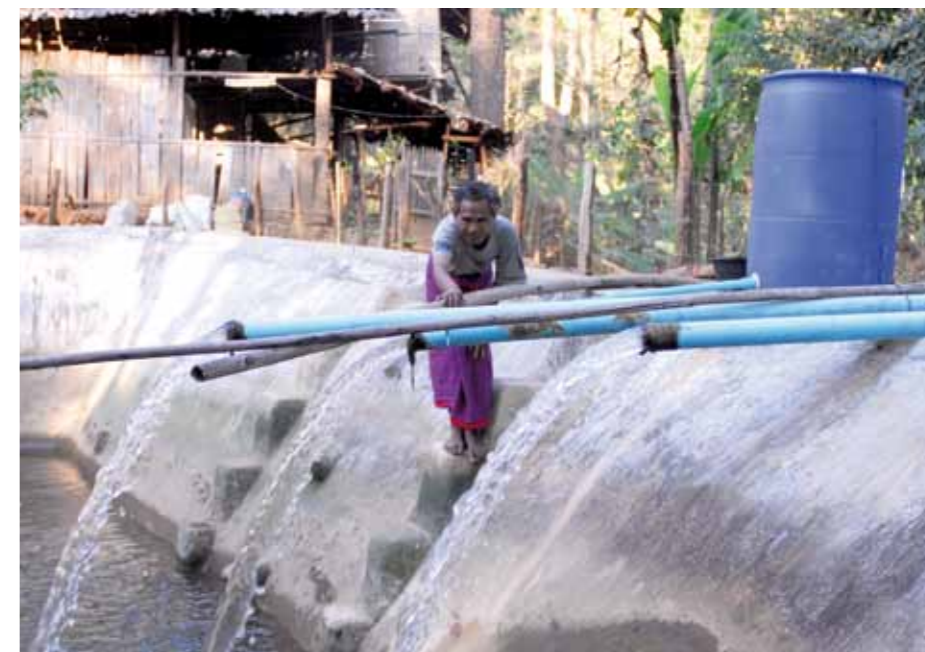
Despite difficult circumstances in the camps, Malteser International was able to assure safe water supply by building rain water collection stations.
